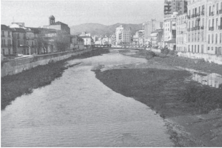
Plate 9.2 The aggraded, embanked channel of the Rio Guadalmedina at Malaga, Spain, in 1980. Sand and gravel brought down from the mountains have raised the bed of the confined channel above the level of the adjacent streets, so putting adjacent buildings at risk of flooding.
