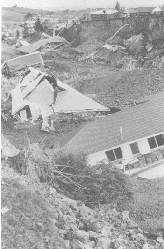
Plate 6.2 Destruction in the suburb of Abbotsford, caused by the block slide of 8 August 1979 (photograph: Bill Brockie).
