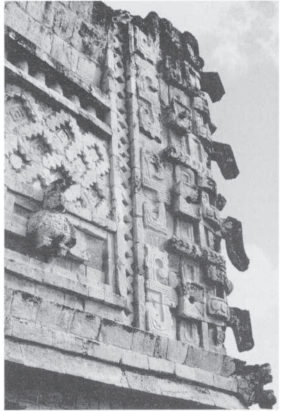
Plate 3.1 Damage due to acid precipitation on the 'Nunnery', part of the Mayan complex at Uxmal, Mexico (photograph: Dr M.D. Turnbull).
