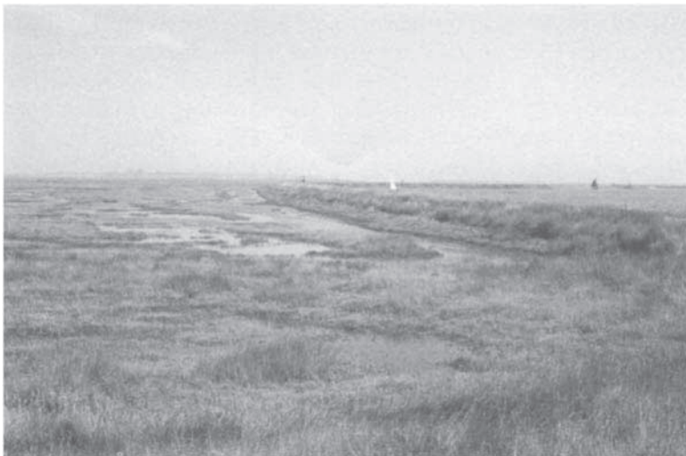
Plate 8.2 Managed realignment of an estuarine shoreline: Tollesbury Fleet, Blackwater estuary, Essex, England. The view is bisected by the now breached old seawall defence line. To the left foreground, natural salt marsh is just being flooded by the rising tide. To the right in the distance, small boats have sailed through the breach into the lower, already well-flooded managed retreat site (photograph: T. Spencer).
